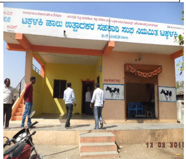
KMF AI Center Takkalike, Vijayapura Taluk
